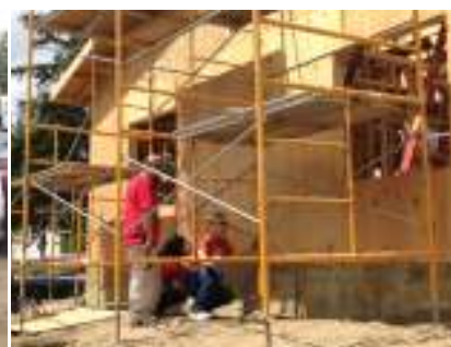
Target team hard at work on Rayton home in Virginia
